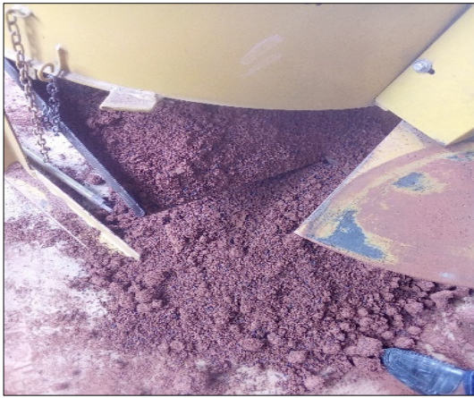
Fig 6: Mixing solid waste material with laterite
